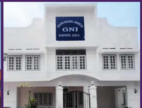
National Indonesia Building Gresik ( 2022 )
