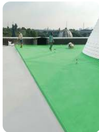
Dak Beton Masjid
