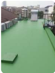
Dak Beton Rumah & High Rise Building
