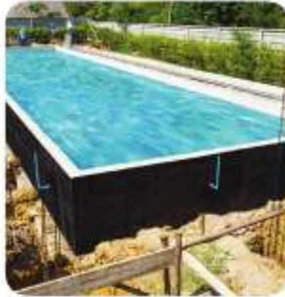
Outerwall of Swimming pool
