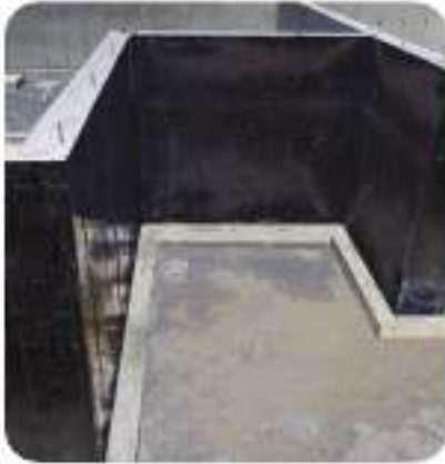
Outerwall of Basement
