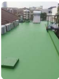
Dak Beton Rumah & High Rise Building
