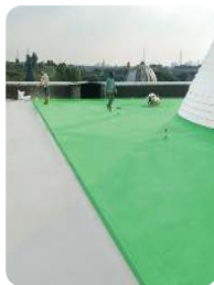
Dak Beton Masjid
