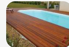
Wooden Pool Deck
