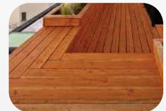
Wooden Park Deck
