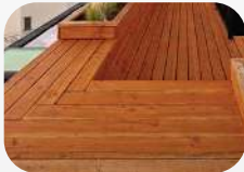
Wooden Park Deck
