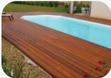
Wooden Pool Deck
